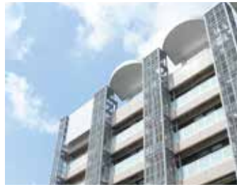
16 Comprehensive Research Building
