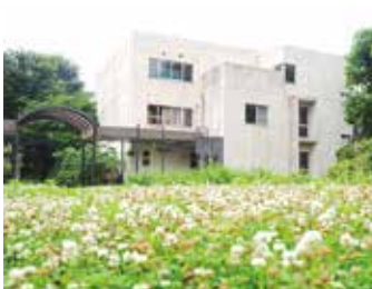
10 Student Club Facility
